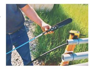
Use of a MaxCell Rodder Head can facilitate placement of MaxCell innerduct. When the "Paddle" exits the conduit run, MaxCell should be half-hitched with pull tape to the rodder head (after removing retaining screws and PVC paddle from the clevis/rodder head assembly). The clevis assembly itself is on a swivel which prevents any twisting or kinking of MaxCell during installation.
